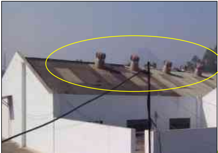
3% Energy Saved by Air ventilators installation
