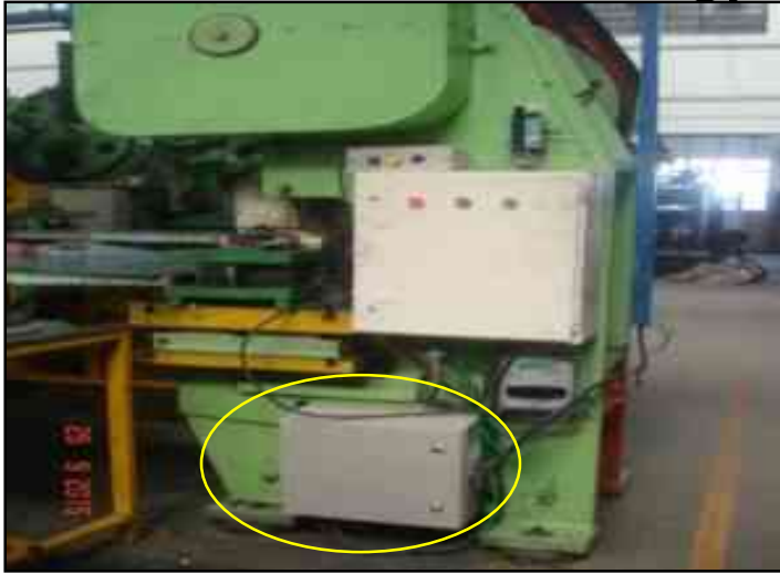
30% Energy Saved by instillation of VFD's
