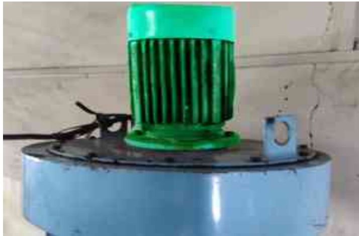
Powder Recovery Blower Motor (3 HP )
