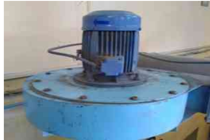
Powder Recovery Blower Motor (2 HP )
