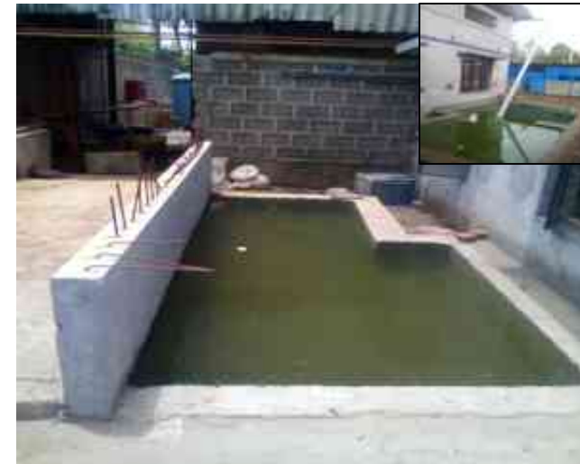
Rain Water Harvesting Tank (capacity 10 kl) Near Compressor Room
