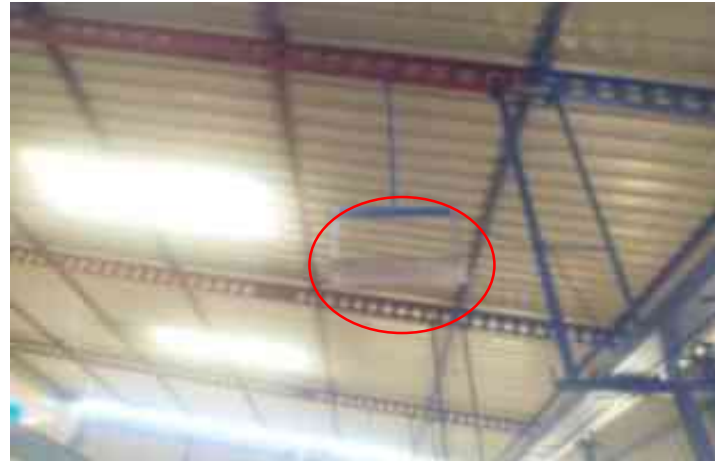
Replace CFL by LED(870Watts)
